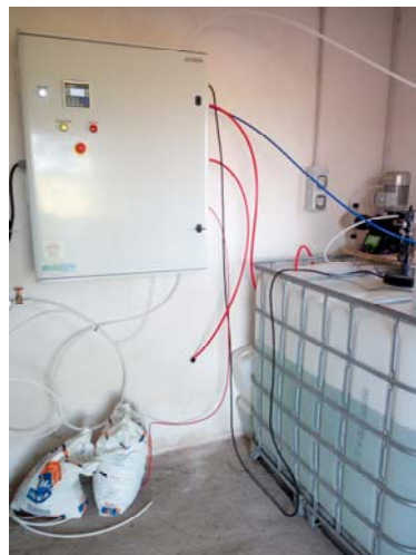
Unit ELA2000HD with brine and Anolyte tank and dosing pump
