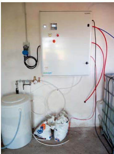
Unit ELA2000HD with brine and Anolyte tank and dosing pump
