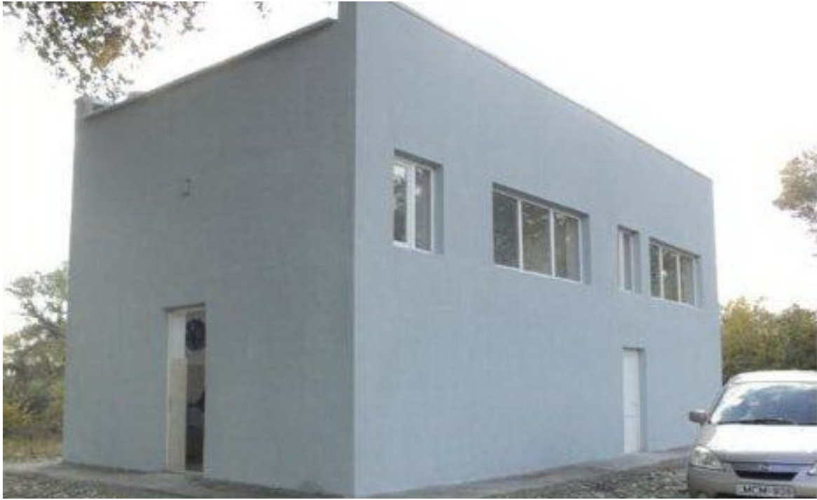
Water purification station
