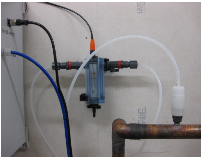
Redox cell and injection point
